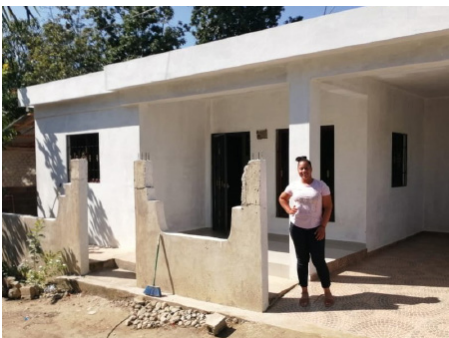
ADOPEM's Eco Vivienda loan in the Dominican Republic enabled this beneficiary to rebuild her house.
